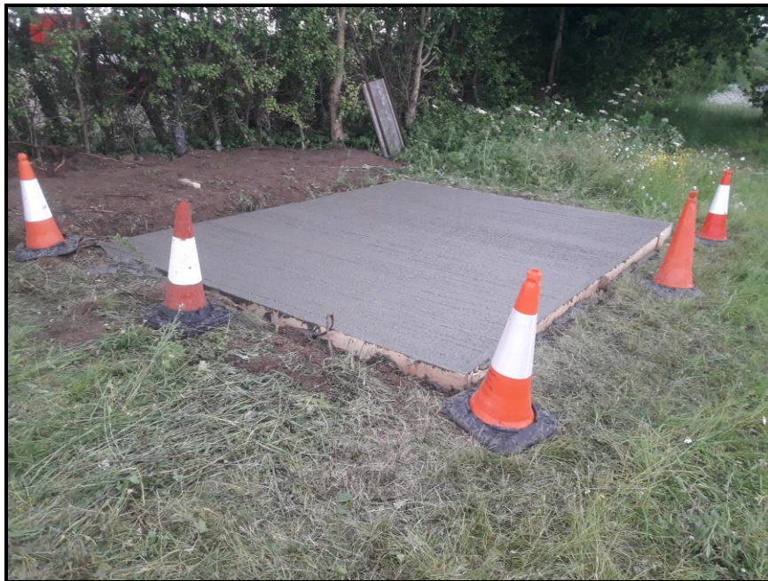
13 th June 2022. Plinth formwork built and fixed to sub base slab.
