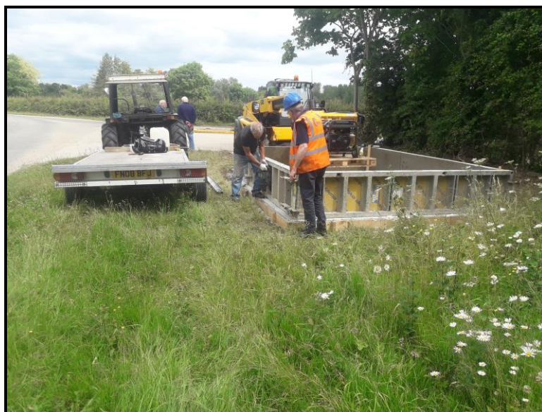
13 th June 2022. Plinth formwork built and fixed to sub base slab.
